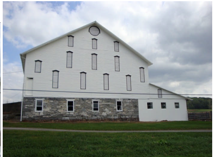
Lane side of the barn.
